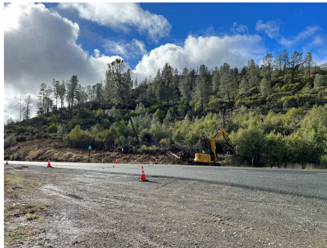
After: SLFPD excavator working along Hwy 29 south of Middletown, CA.
