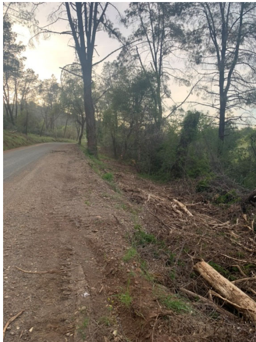
After: Post-treatment with masticator on Jerusalem Grade Road, Middletown, CA.
